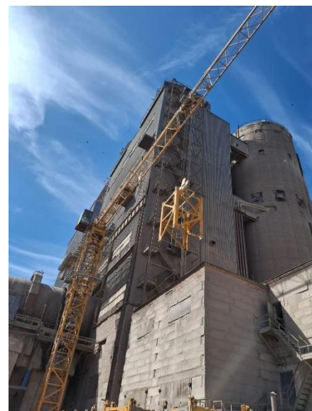
New crane for Line 6 preheater tower
